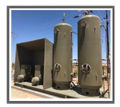
Our simple, reliable and scalable packages are readily available and designed to deliver between 25 and 100 cfm of clean, dry, compressed air.
